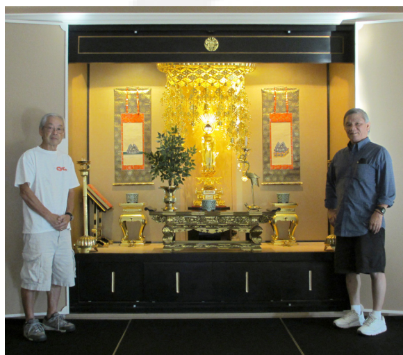
At left: During the months of September and October, Mr. Richard Kagawa and Rev. Peter Hata completed their project to illuminate the temple's altar in preparation for the 2013 Hoonko Service. The altar itself, completed in 2009, is the work Mr. Arne Hansen, with support from Mr. Roy Higa and of course, Rev. Ken Kawawata. This 2013 project involved several tedious but necessary preliminary steps. However, the fruits of their labor are shown in the photo at left (the overhead lighting in the hall was off for this photo). Not only are the scrolls of founders Shinran Shonin and Rennyo Shonin much more visible, the gohonzon or central object of reverence, Amida Buddha — the symbol of infinite wisdom and compassion — is radiant.
